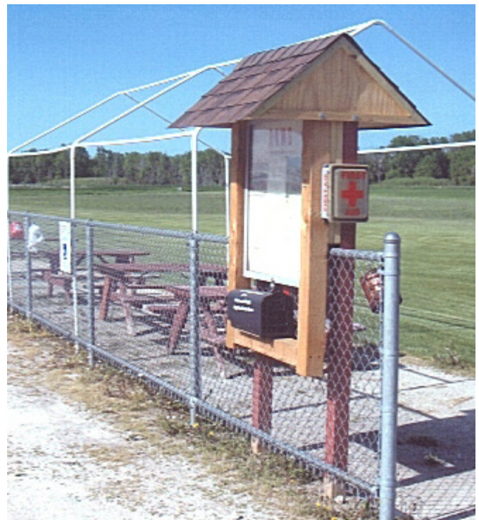
Above: Rebuilt frequency board (side away from camera) and bulletin board, as relocated southerly along east fence line. Framework for another sun shade, donated by Dell Fisher, also shown. NOTE new side post location of Emergency Kit (eye level).
