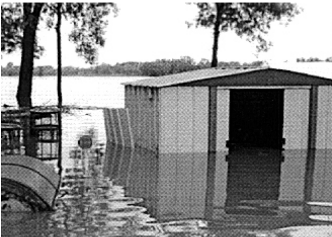
View N, flood on roller, and rake shed doorlocks
