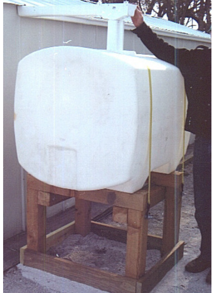
Above: 60 Gallon rain cistern tank installed between sheds by Bill Geipel, Brian Lorentzen & Bob Kabella, to the right.
