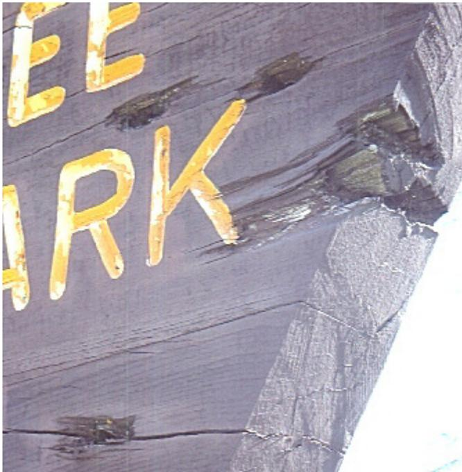
*Above: The "exit wound" holes made by 4 of the 5 bullet holes show here on the west face. Mel, a retired professional wood worker, will custom make wood plugs. The peeling of the yellow routed lettering, revealing the white primer base in both photos, will also be addressed.*
